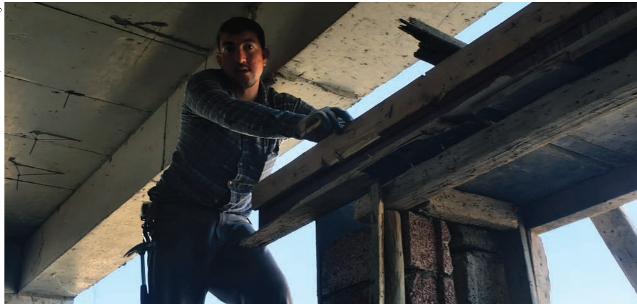
An IDP carpenter trained by an ACT member also received a grant to start a business. Here he is shown working on the alignment of concrete beams ready for casting in Duhok.
