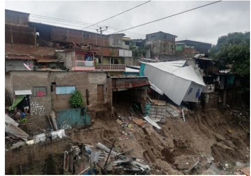
Figure 1 San Salvador. Precarious settlements were heavily damaged by the storm.
